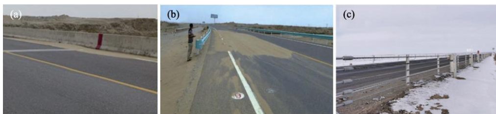
Fig. 1 Sand deposition near the guardrails of desert highways. (a), concrete guardrail; (b), W-beam guardrail (Li et al., 2016); (c), cable guardrail.
